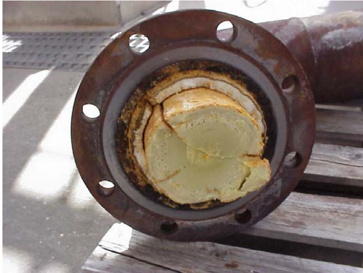
Figure A-4. Vent line obstructed by polymer layers.
