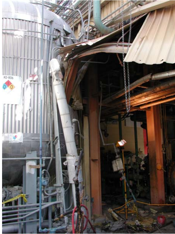
Figure 5. Damaged girder.
