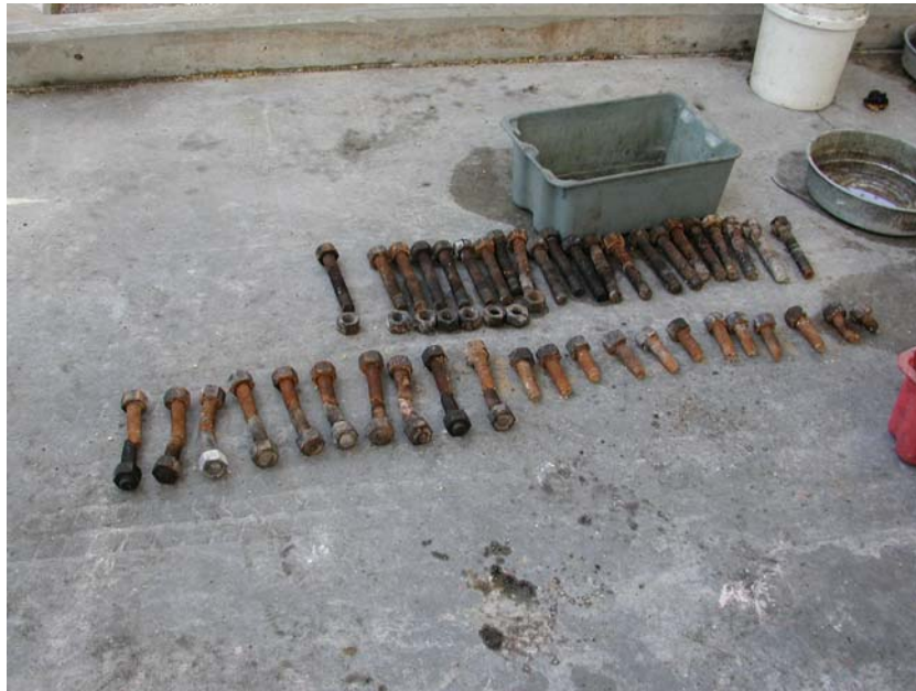
Figure A-2. Failed bolts from polymer catch tank cover.
